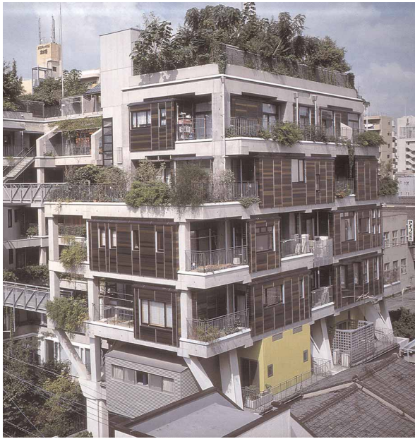
Figure 2 Corner view of the Osaka Gas experimental housing project NEXT21 (1994). Yoshitika Utida, chief architect, and colleagues note the public roof garden and small private 'gardens' as part of the units. Note too the anodized aluminium facade system which allows adaptation to the interior layout of the units; the panels can be dismantled from the inside without exterior scaffolding. Photograph: Osaka Gas.
